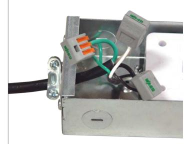
2) With power off at the breaker, feed power leads through strain relief and cover plate and secure.
